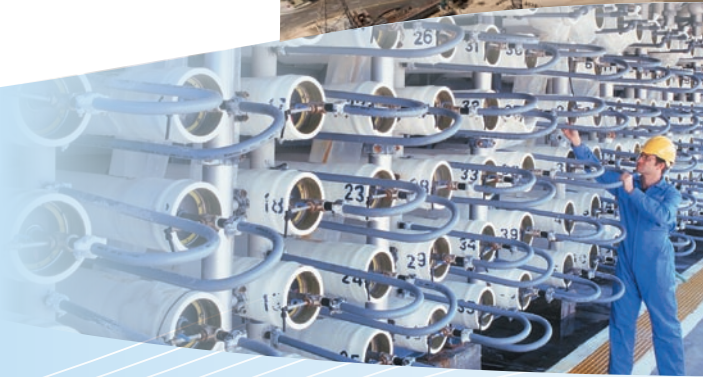
Larnaca SWRO 21.5 million m 3 /year BOT project, operating since 2001 in Larnaca, Cyprus
