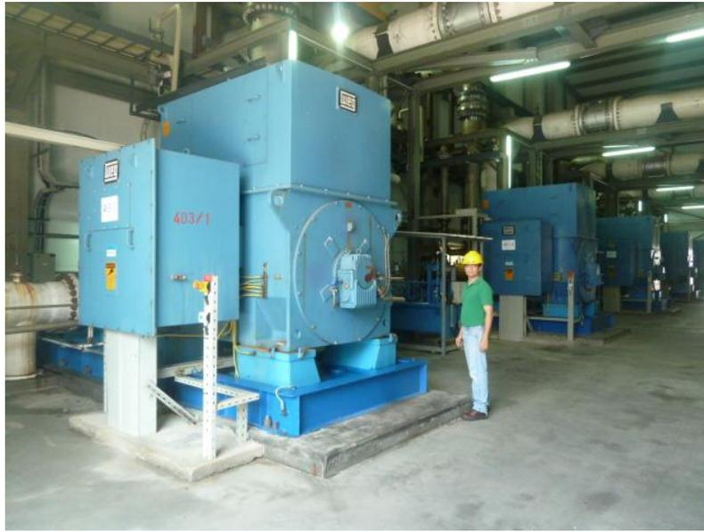
**Figure 4: High Pressure Pumps**
